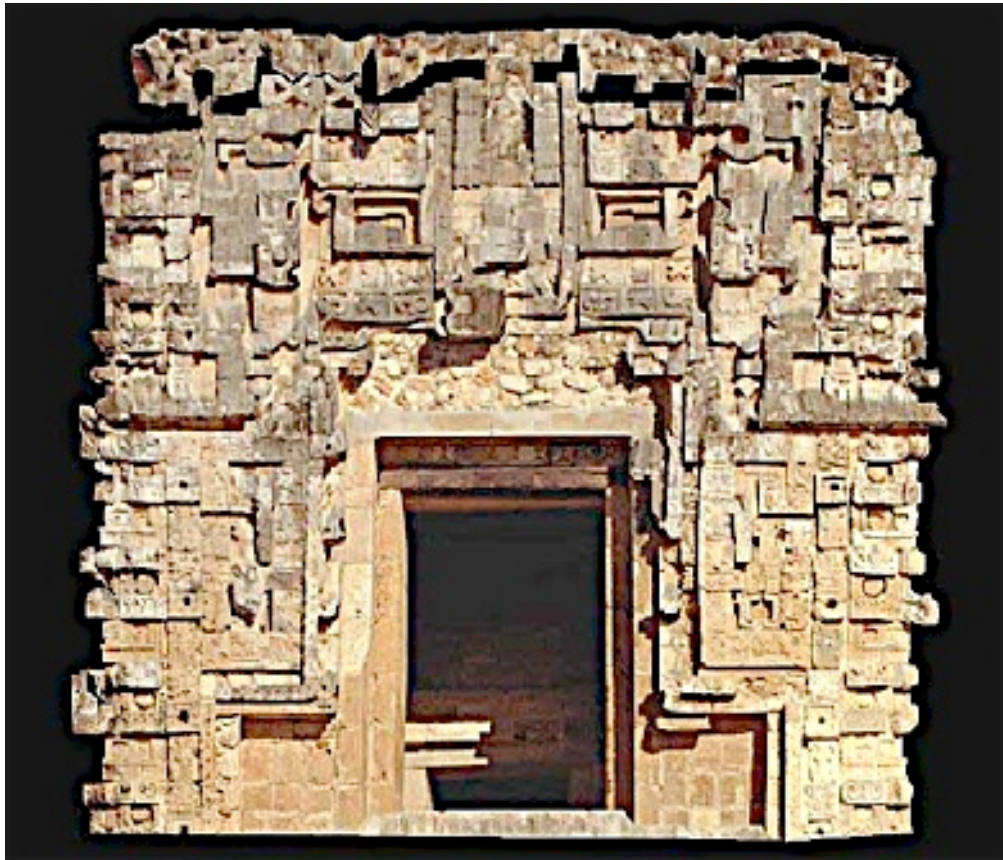
Figure 15. Orthophotograph of the Chenes Temple (AD 800-1000) on the west side of the Adivino Pyramid from which scaled drawings can be made. 1999. Orthophotograph by Michael Clowes.
