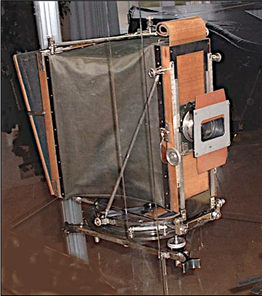
Figure 12. Albrecht Meydenbauer's photogrammetric camera, c 1880. Pic: Paul G. Bryan, 2001.
