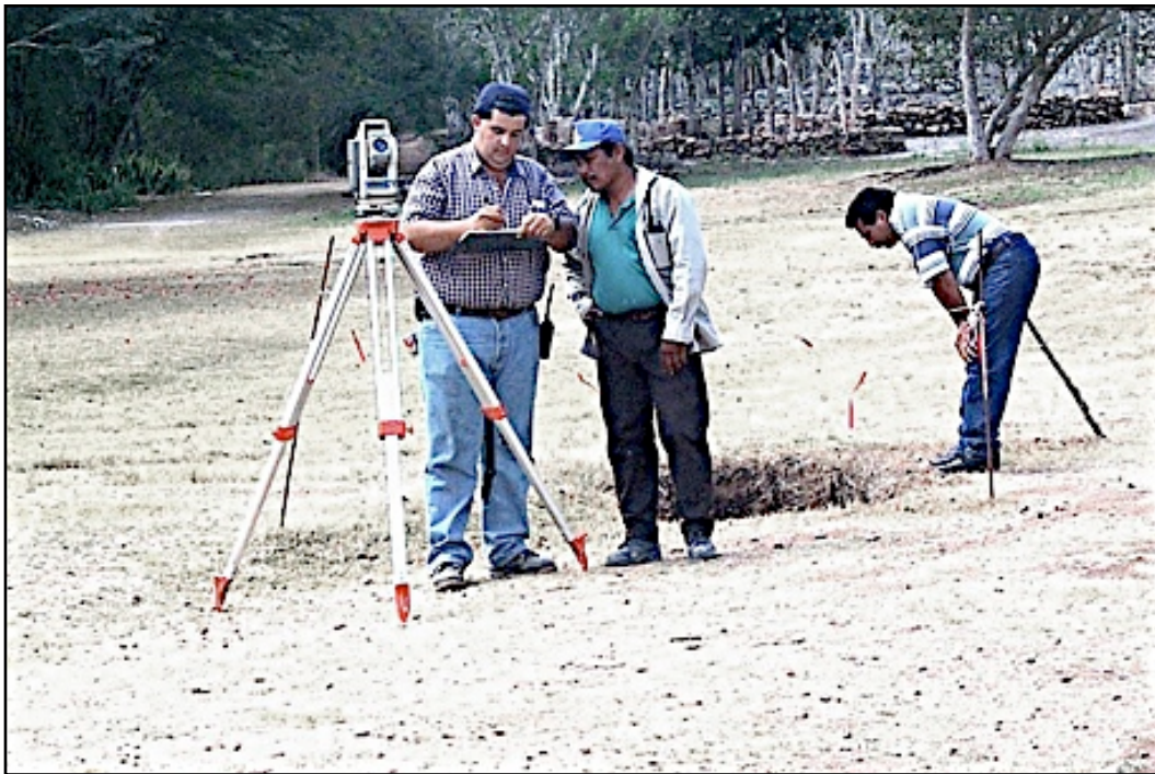
Nikon total station used for acquiring the 3-D coordinates of survey control targets on the pyramid. Engineer Francisco Mendoza d'Argence surveying. Pic: Roberto Centeno Lara. 1999.
