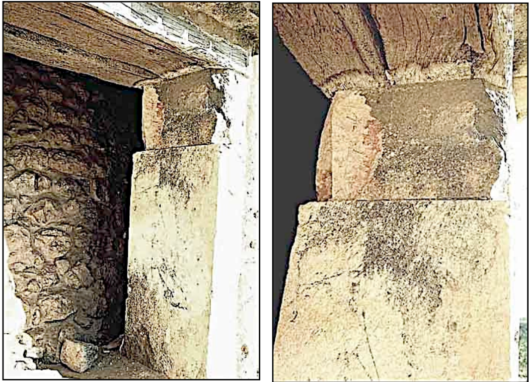
Shearing of stone due to downward thrust of pyramid onto wood lintel. Pic: L. G. Desmond. 1989.
