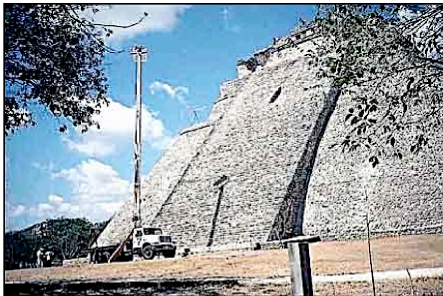
Adivino Pyramid east facade Hydraulic lift used to photograph the upper east, south and north facades of the pyramid. Bryan and Clowes are making stereo 3D photos from the lift bucket. Pic: L. G. Desmond. 1999.
