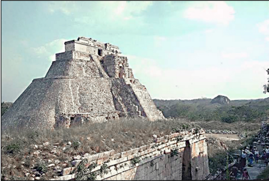
Adivino Pyramid from the northwest. Note vertical cracks in west facade filled with concrete. Pic: Lawrence G. Desmond, 1990.
