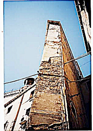
Photo 10. Apartment building buttress.
