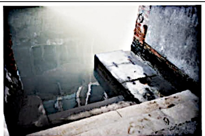
Photo 31. Boat landing under the Ponte de la Malvasia Vecchia, south side of rio della Verona, as a potential instrument platform. New laser theodolites can be used effectively in very constricted locations such as shown in this photo and Photo 30.
