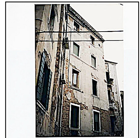
Photo 4. Apartment building to the east of Fenice Theater.
