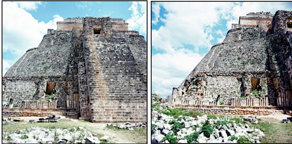
West facade of the Adivino Pyramid, Uxmal. 3D stereo used for photogrammetric processing. Pic: Desmond, 1990.
